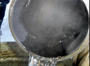
Two months after the HydroFLOW 120i was installed - Hard scale is not accumulating on the area that was cleaned after the first inspection. Existing scale can be easily flaked off.
