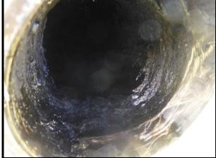
One week after the HydroFLOW 120i was installed - The scale was much softer and easily removed with a knife. A ring was cleaned in order to determine if scale will not accumulate on a clean surface as long as the 120i is in operation.
