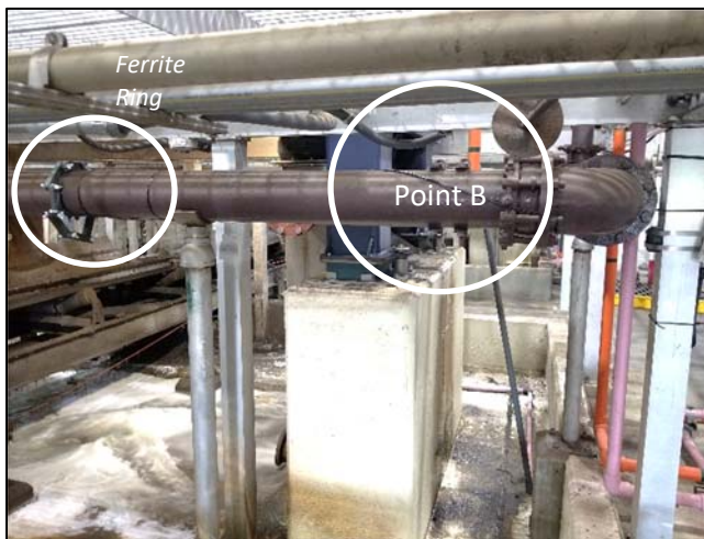
Figure 2: Second Ferrite Ring / Polymer Injection, Point B
